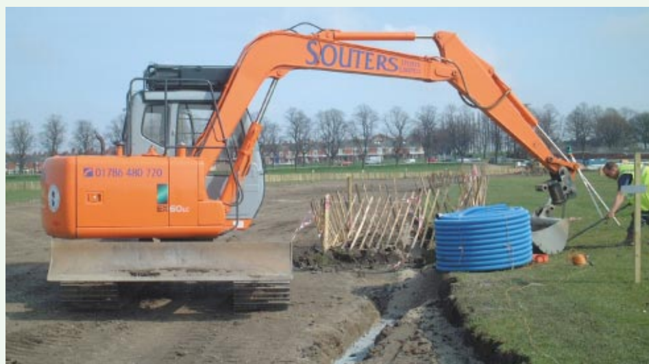
Construction works include primary drainage.
